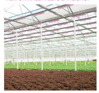
With a light output of 860  $\mu$ mol/m<sup>2</sup>.s and a system efficacy of 2.7  $\mu$ mol/J, the HortiLED TOP delivers optimum performance and energy savings.
